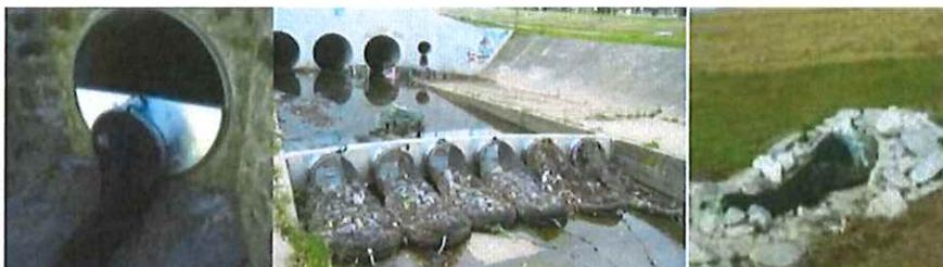
Filets sur exutoires (<http://stormwatersystems.com/stormx-netting-trash-trap/>)
